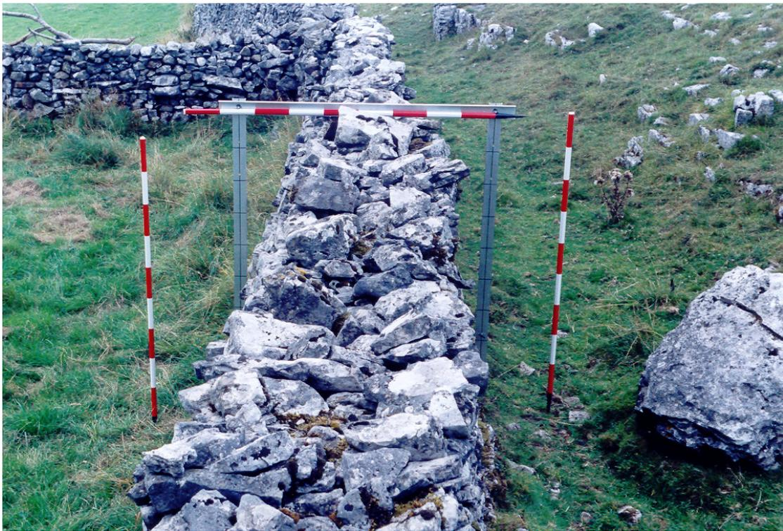
**Part of the medieval infield boundary wall at Winskill built *circa* 1300. This double wall was made wider than normal to accommodate large blocks of limestone quarried from the adjacent scar. The original topstones would have been laid flat, and made to project on the outside edge of the wall, the side on the right, to prevent wolves jumping into the infield.**
